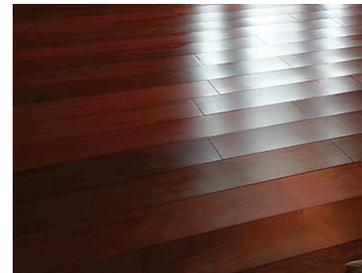
Wood that loses too much moisture can gap. Gapping occurs between floor boards. Gaps can vary in size and are considered normal if they appear and disappear during seasonal changes in humidity. Both of these issues can be minimized by maintaining an environment that is consistently between 60-80 degrees Fahrenheit, and 30-50% humidity. Significant fluctuations outside these ranges can result in cupping or gaps.
